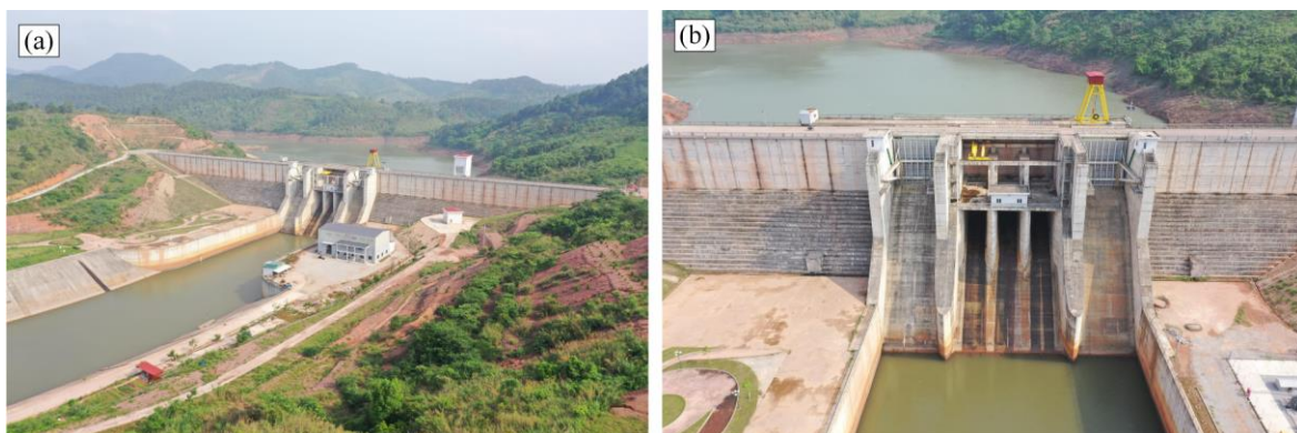
Figure 1. The Ban Lai dam after construction: (a) Perspective view and (b) Front view
